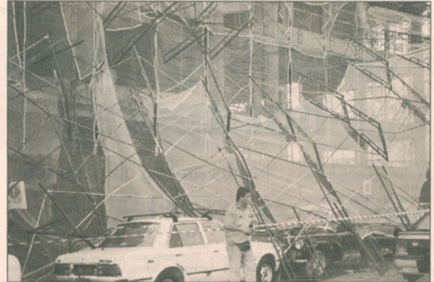
ABOVE: The fallen structure in Puchong
