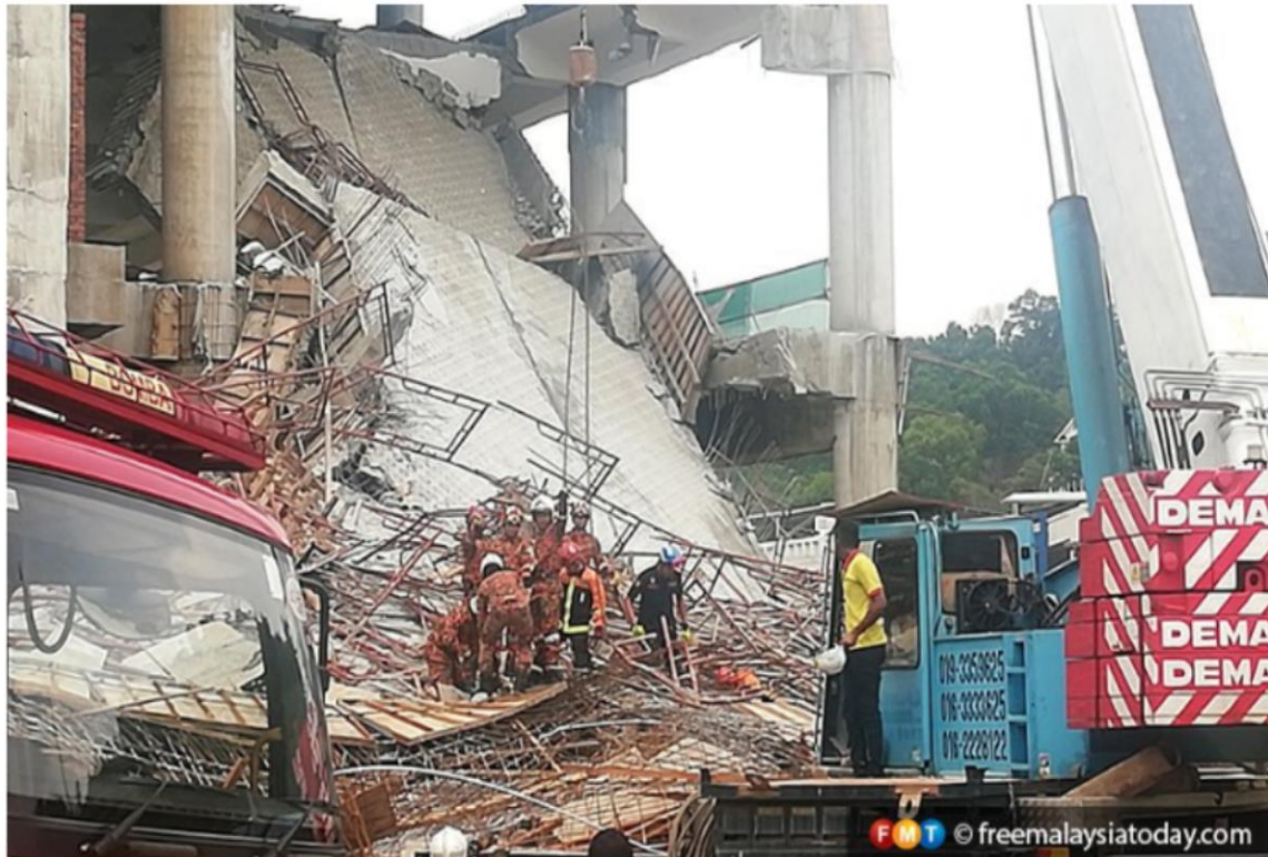
An Indonesian couple, working as construction workers, were killed when a building collapsed near the Gombak LRT station on May 23.
