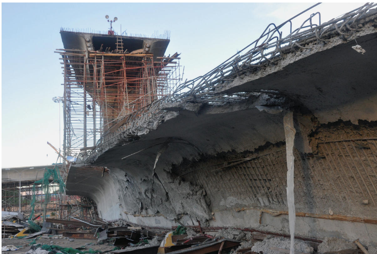
Photo 1.0: Front view of the scene showing collapse of supporting false work structure for Batu Maung Interchange work, Penang Second Bridge project
