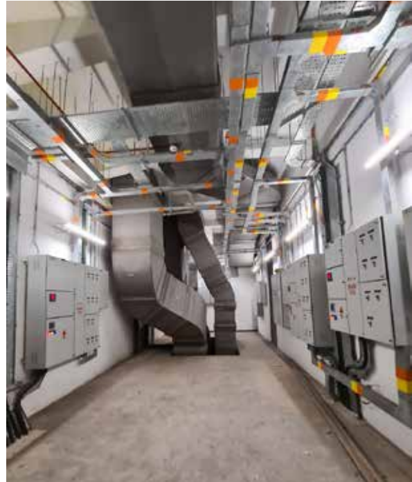
Figure 9: The new electrical sub-switch boards
