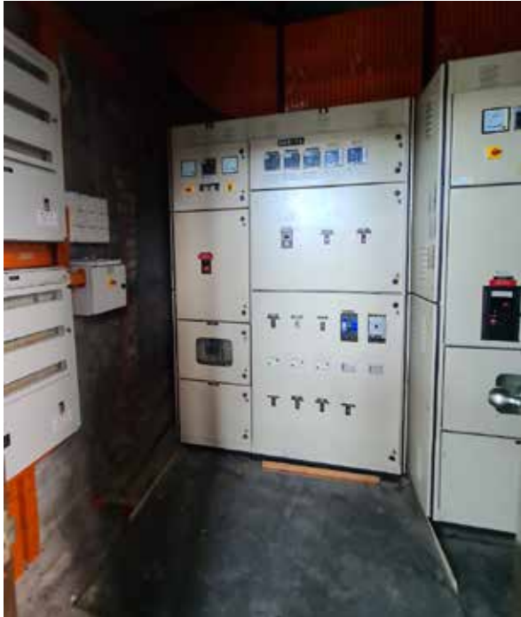
Figure 9: The new electrical sub-switch boards
