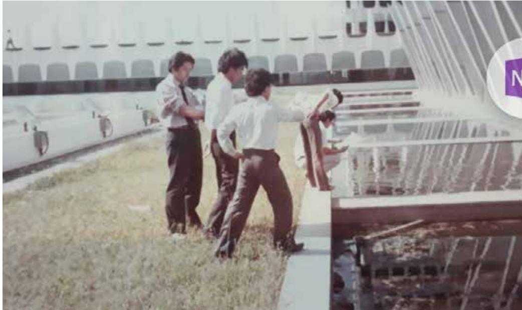
Figure 12: View of pool and grass area at the lower rooftop in 1987
