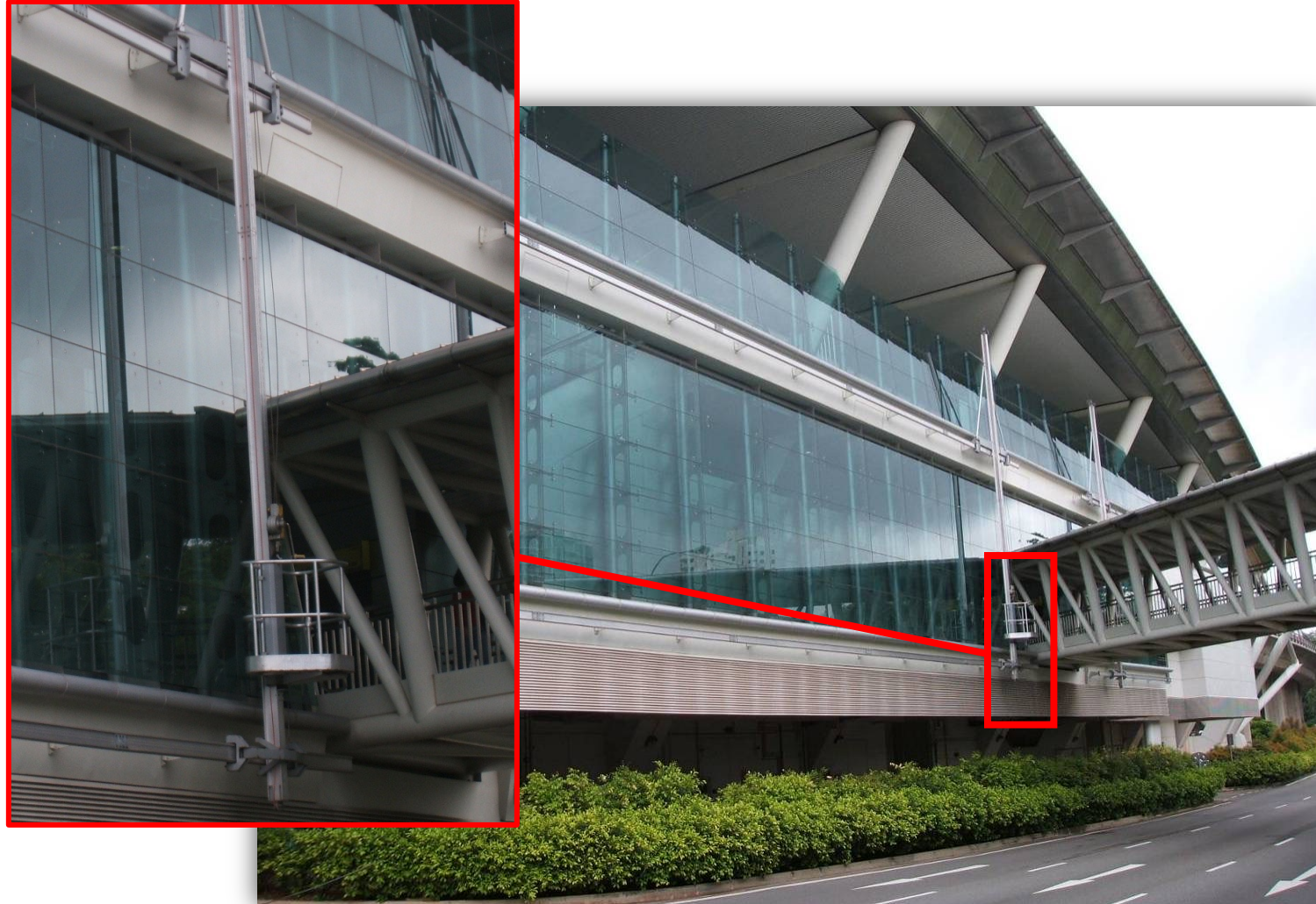
Dover MRT Station with permanent maintenance gondola
