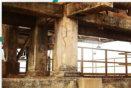
Failing Fireproofing (SCE Element)
