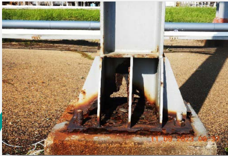
Severely Corroded Structure Supporting Flare Line
