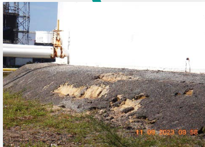
C1 Tank Foundation damage due to degrading asphalt
