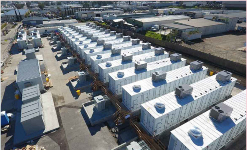
Typical utility-scale BESS. Source : Energi Media
