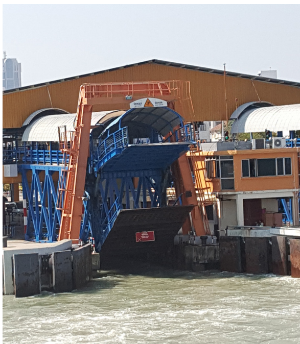
Photo 5: For old ferries system, docking platforms were mounted at the terminal. Passengers used the upper platform and vehicles used the lower platform.
