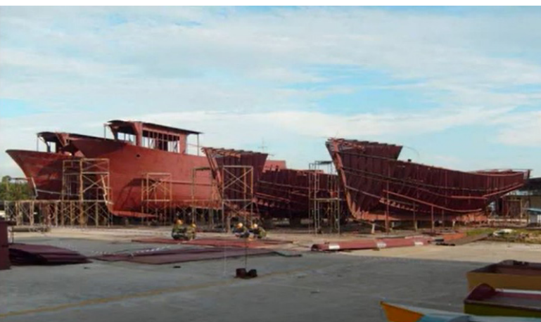
Steel purse seiners and trawlers being built at UniKL MIMET in 2008.
