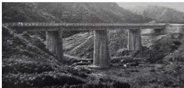
The new completed Sungai Bertam Bridge, Cameron Highlands in 1962.
