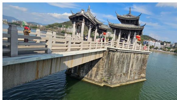
View of a stone pier with an arrow-shaped upstream face designed to deflect the oncoming current and reduce structural stress. The granite beam rests directly atop the pier.
