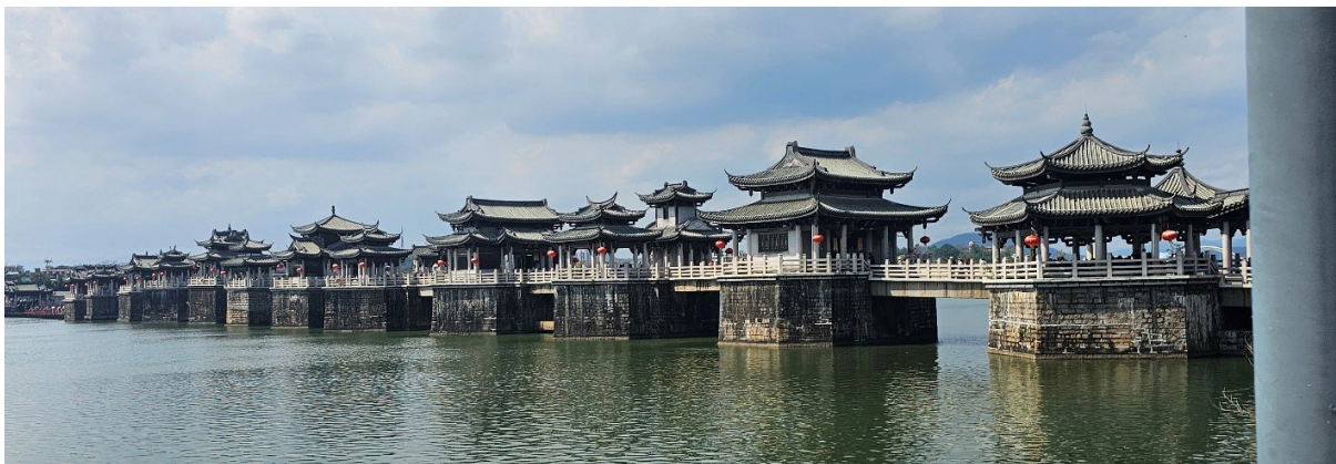
View of the bridge from eastern bank of Han River.
