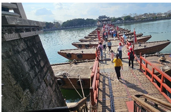
View of the middle section of the bridge where pontoons link the two ends of the stone-pier decks.
