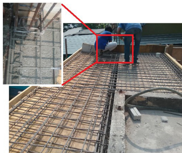
Figure 5: Part of the enlarged section and casting of LWAC.
