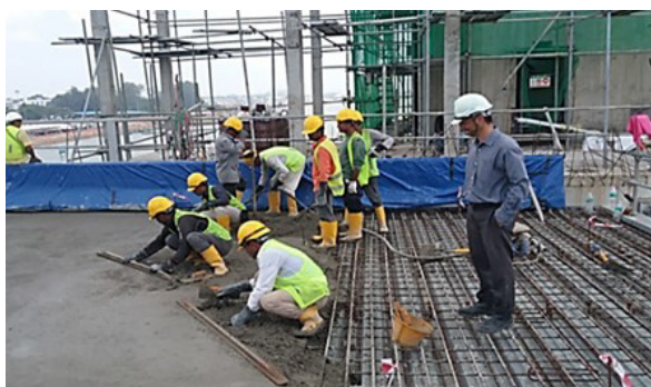
Figure 3: Workable lightweight aggregate concrete on the bascule (top) and pedestrian (bottom) of Terengganu Drawbridge
