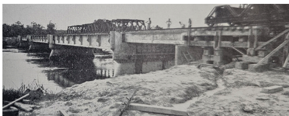
Launching of prestressed concrete beams using PWD labour force
