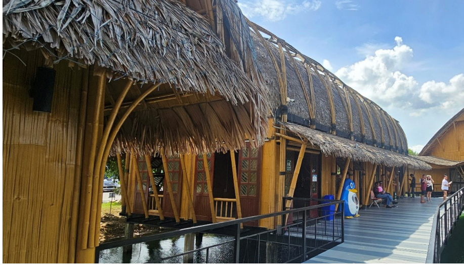
The bamboo roof truss, skillfully crafted and finished with Palmyra palm fronds, combines creative artistry with sustainable design.
