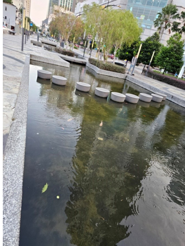
Photo 1: Part of walkway at the upper reach of Jalan Wong Ah Fook is a shallow channel on a concrete slab.
