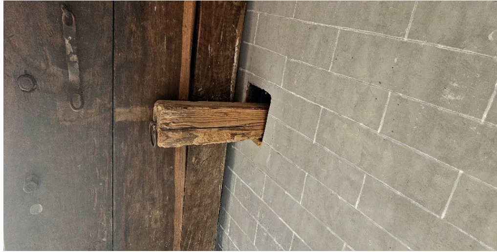
Figure 11: Left: The 120mm thick hardwood timber door with a 10mm thick steel plate. Right: The 200mm timber bolt that can be slid from one side of the wall to a hole on the opposite side to prevent forced entries.
