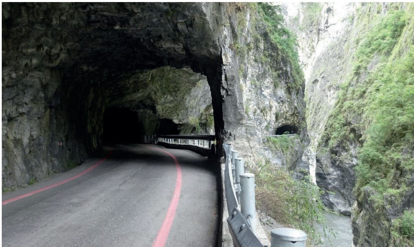
Picture 1: Narrow part of the Taroko Gorge Highway
