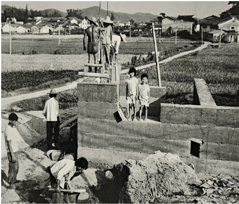
Figure 1: Archive photograph showing the timber formwork used for ramping the earth-mixture to make the walls
