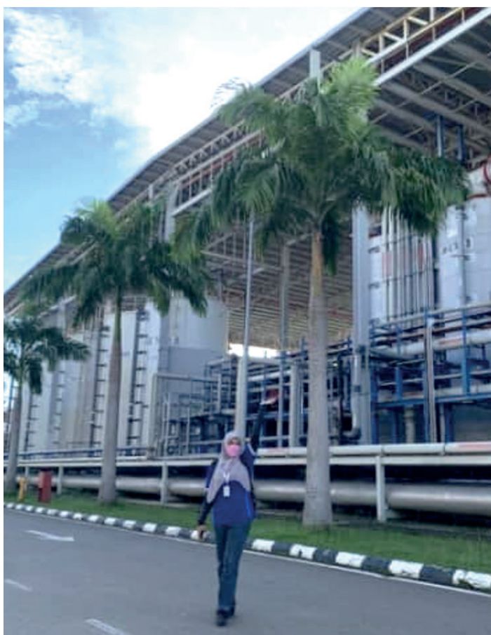
Open structure WWTP
