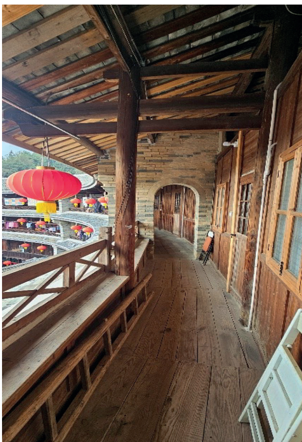
Figure 10: View of a firewall made of bricks. The timber floor is also tiled for sound insulation as well to protect the floor boards in case of fire
