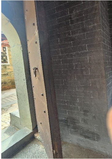
Figure 11: Left: The 120mm thick hardwood timber door with a 10mm thick steel plate. Right: The 200mm timber bolt that can be slid from one side of the wall to a hole on the opposite side to prevent forced entries.
