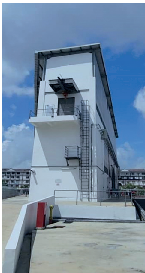
Closed structure WWTP
