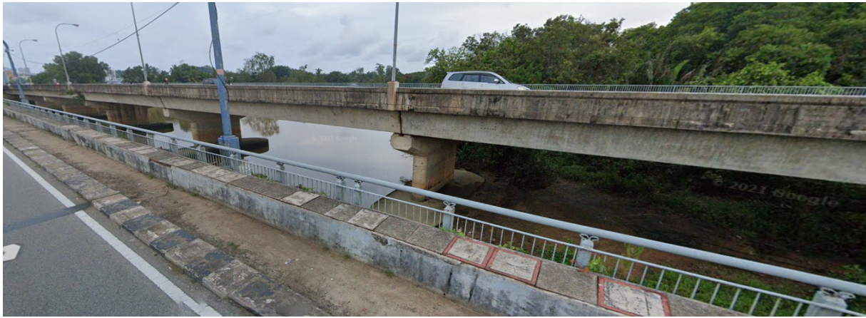
Present view of the bridge
