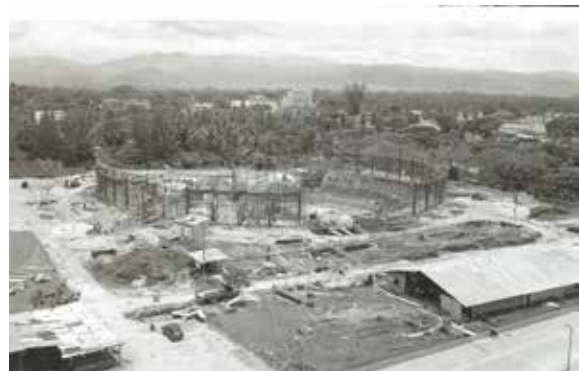
Stadium Negara under construction in 1961. Construction works for the 10,000-seat Stadium Negara commenced in 1960 and was completed in 1962 at the cost of RM34 million. It was the country's first indoor stadium as well as the best indoor stadium in South East Asia then and was listed as a National Monument under the National Heritage Act, 2005.
