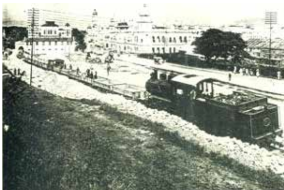
Train used in construction of Victory Avenue. The Federal Court Building in the background constructed with bricks transported by trains from Brickfields.
