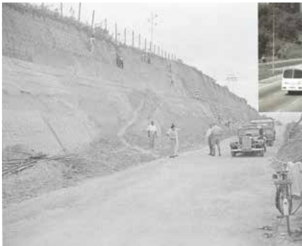
Photo taken on 29.9.1958 showing the Minister of Works, Posts and Telecoms, YB Tun Sarbon bin Jubir (with coat and songkok) walking to an engineer on the dual-carriage way construction beginning from Bangsar Road to the Sungei Way traffic roundabout. The road was opened on 14.1.1959 by the Minister of Works, Posts and Telecoms.
