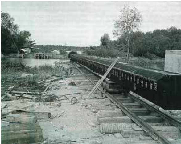
Batu Pahat Bridge under construction March 14, 1966
