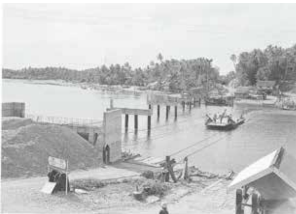
The Marang Bridge was one of the bridges constructed in 1964 by the Public Works Department, or JKR, in Terengganu. This was to replace the ferries operated by them at the Kemaman, Dungun, Losong and Marang districts. The then Marang ferry used a motorised cable pontoon system (see photo). It was the only river crossing on Federal Route 3 running along the east coast of Peninsular Malaysia.
