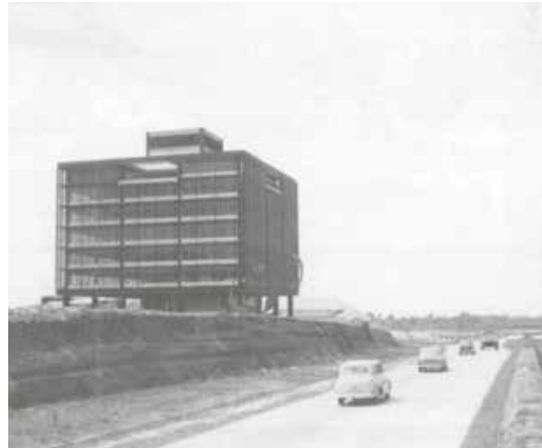
The Federal Highway, Kuala Lumpur-Port Swettenham Highway started construction in 1956 and was completed in 1959 at the cost of RM2 million. The highway linked Petaling Jaya and Sungei Way along the route with a designed travelling speed of 60 mph.
