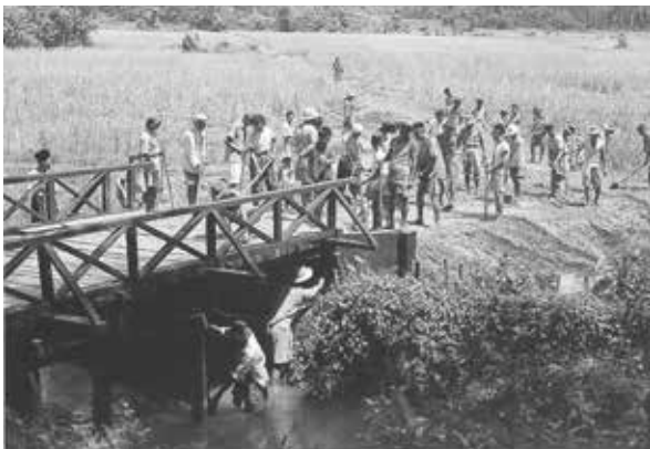
Gotong Royong project of levelling a village road near a bridge by villagers of Kg Seri Rembau, Negeri Sembilan in 1952.
