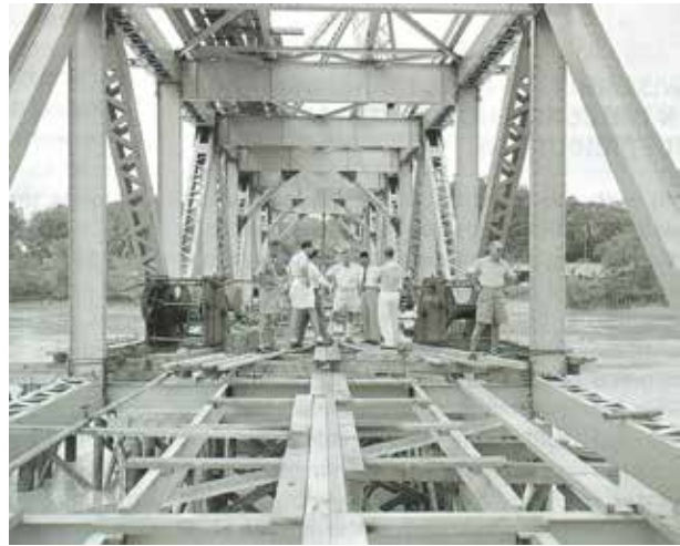
Inspection by engineers at the construction site of Kota Bridge on September 29, 1958.
