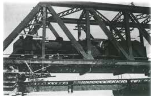
Train passing the railway bridge
