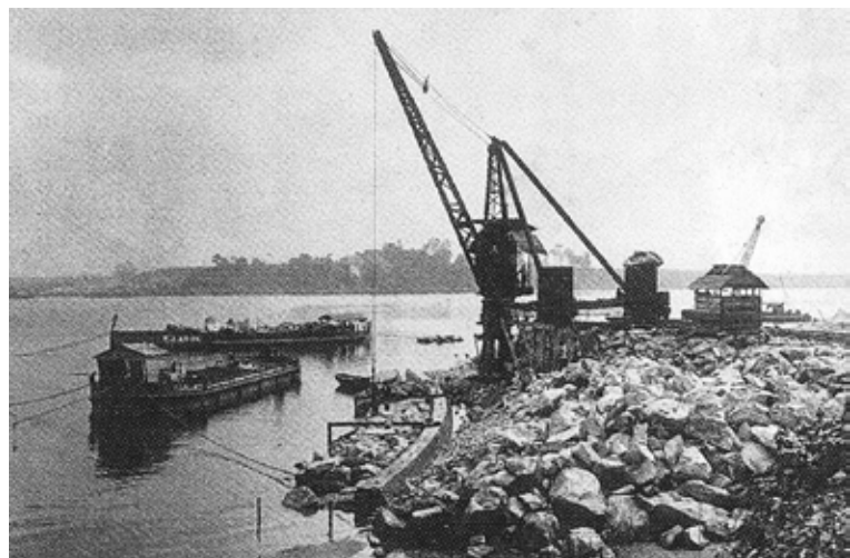
Progress work at south (Woodlands) end of the Causeway in June 1921
