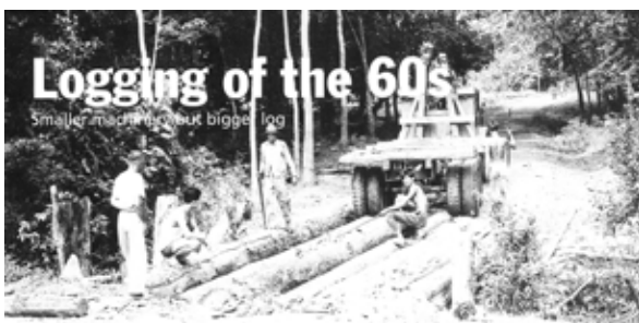
Logging of the 60s – Construction of bridge using timber log.
