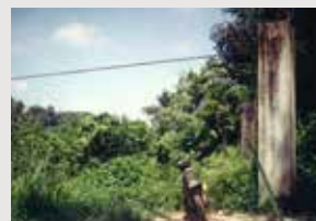
The concrete stump holding the overhead cable that enables the pulley to slide along as the boat crosses the river
