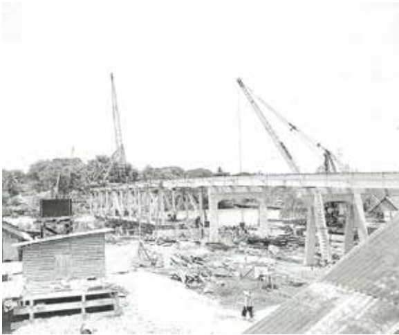
60-year-old Klang Kota Bridge – First Double-Decker Bridge in Malaysia Construction of Kota Bridge in progress September 19, 1958.
