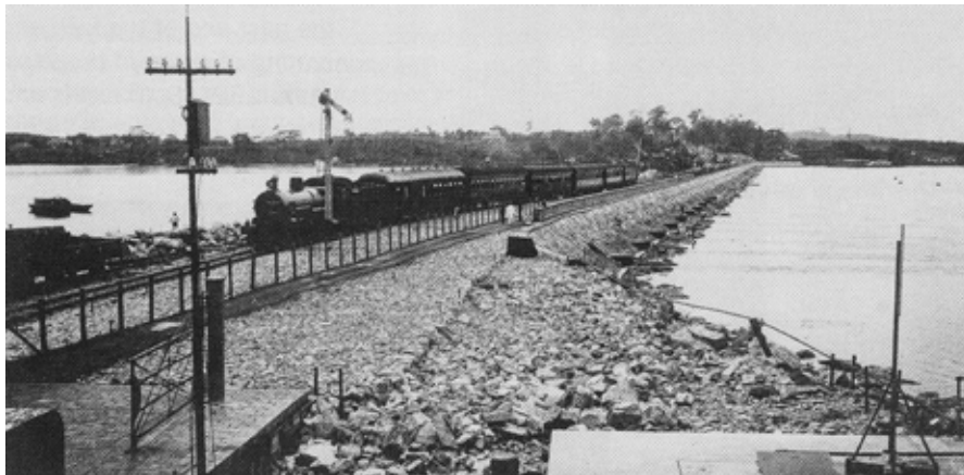
View of the Causeway taken from the operating cabin showing a passenger train from Singapore on the temporary railway track, December 1923.
