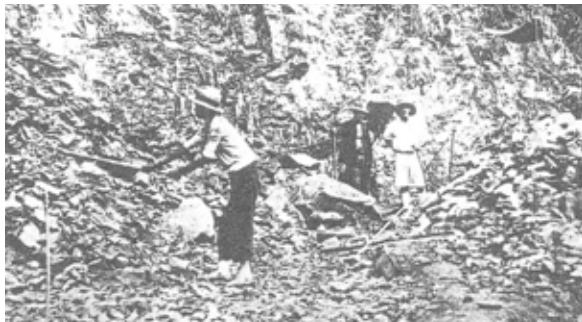
Cameron Highlands road construction in the early days. Note the absence of machinery for the construction of Cameron Highlands road and the dress of an engineer in those days.
