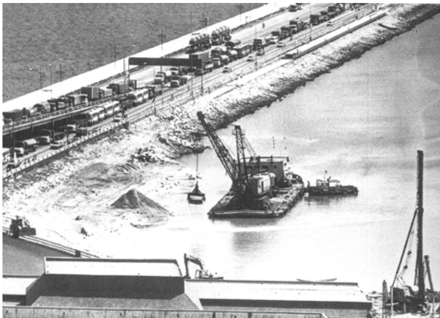
Work in progress to reclaim and widen the Causeway at the Johore end, February 1989.
