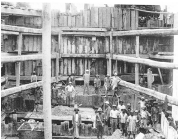
Construction of cofferdam at the east end of the lock and concreting of apron in progress, June 1921. Both locals and Europeans worked together to complete the causeway.
