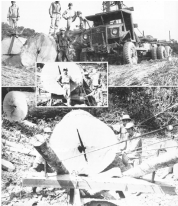
The Lumberjack Team of the 60s - Loading huge log onto jungle timber lorry side way using pulley and winch system.
