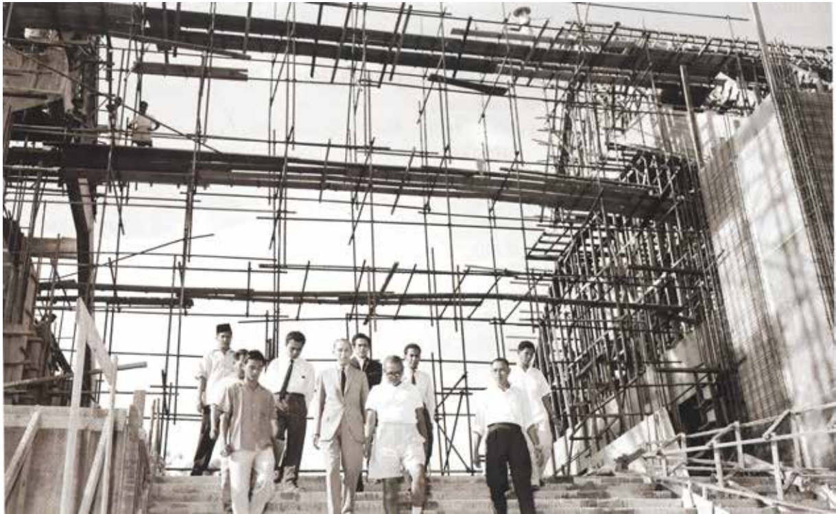
Muzium Negara, under construction in 1962. Tunku Abdul Rahman Putra inspecting the National Museum building under construction in 1962.
