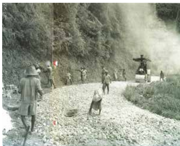
Old Bentong Road upgrading works in 1940s using the old method of macadam road construction. Crushed stones of 100 to 150 mm sizes that were manually laid and rolled with steam roller were commonly used in the olden days. Note the cloud of steam generated behind the roller and the small chimney discharging smoke from burning coal.
