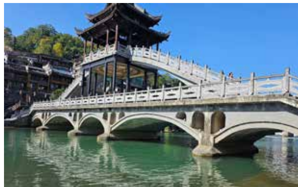
Photo 5: Phoenix Hong Bridge
