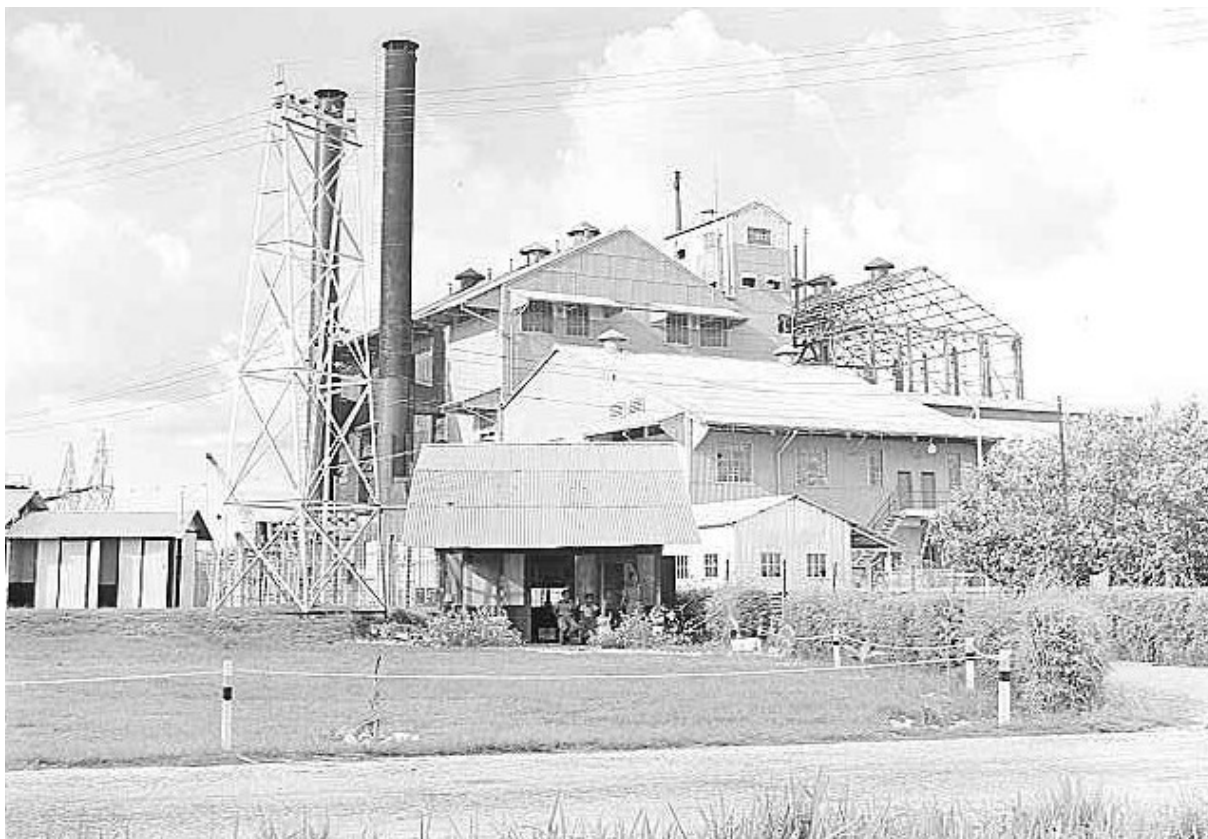
View of Batu Gajah steam power power station situated at Tanjung Tualang taken in 1953. Notice the overhead electric cable connected to the power station through the pylon. A tall chimney was built to emit black smoke from the coal fire boiler to generate steam for electricity generation. (Photo courtesy of Jabatan Penerangan Malaysia)
