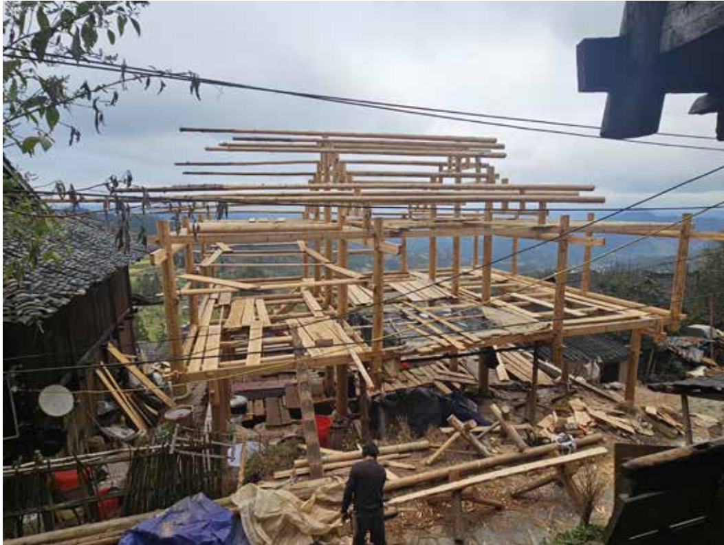
Photo 9: A Miao house being built using traditional methods of construction.
