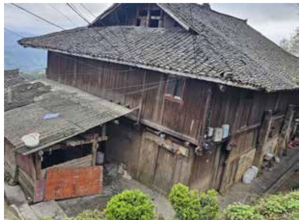
Photo 6: A Miao double-storey house with local fir wood and clay tiles. Notice the ventilation opening at the roof gable.
