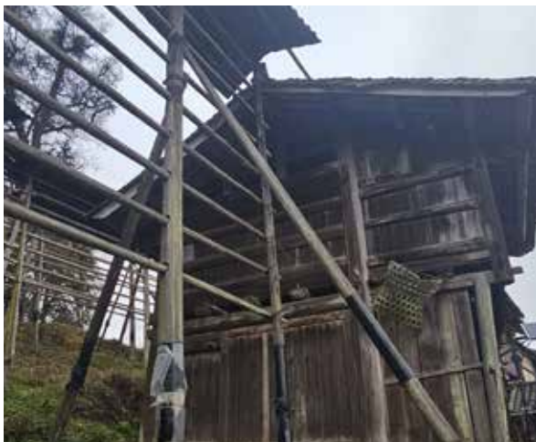
Photo 12: A typical grain drying rack with wooden columns wrapped with metal sheets to prevent creatures from climbing up.
