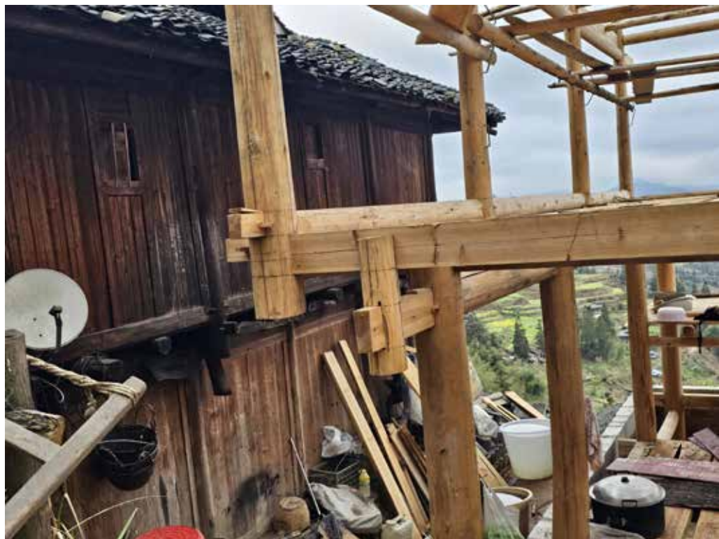
Photo 10: The traditional joinery techniques, without the use of nails, are commonly used by local craftsmen in house construction.
