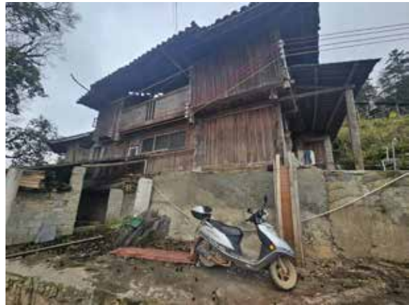
Photo 5: Another typical Miao house construction nestled on a slope.
