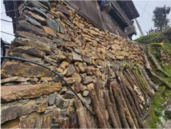
Photo 7: Locally available stones are used as the building's foundation as well as retaining wall.
