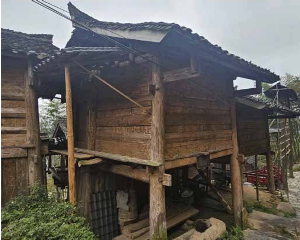
Photo 11: Typical Miao granary stores that store grains on the top level with the ground floor used to store farming tools.
