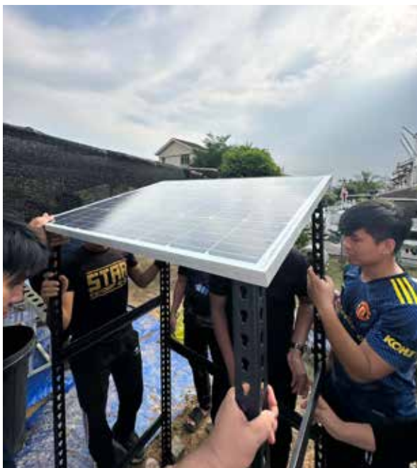
Figure 3: Installation of solar power system.
