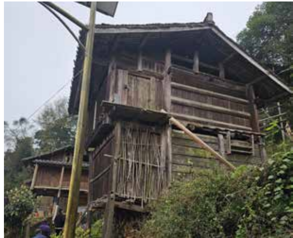
Photo 4: A typical diaojiaolou or stilt house with part of the building extended over the lower slope to gain space instead of constructing an expensive retaining wall.
