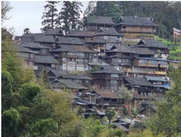
Photo 2: Miao houses are built on stilts on hill slopes. Materials used are mainly local fir timber and clay or timber shingle roofs with masonry foundations.
