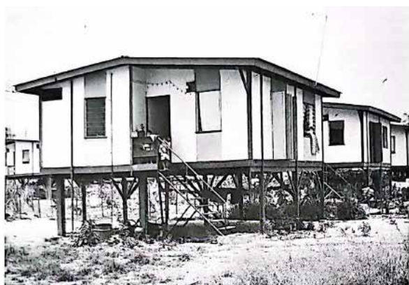
Photo 1: "Factory pre-cut for site assembly modular system" house assembled at Likas Bay, Kota Kinabalu in the 1970s as part of a low-cost housing scheme.
